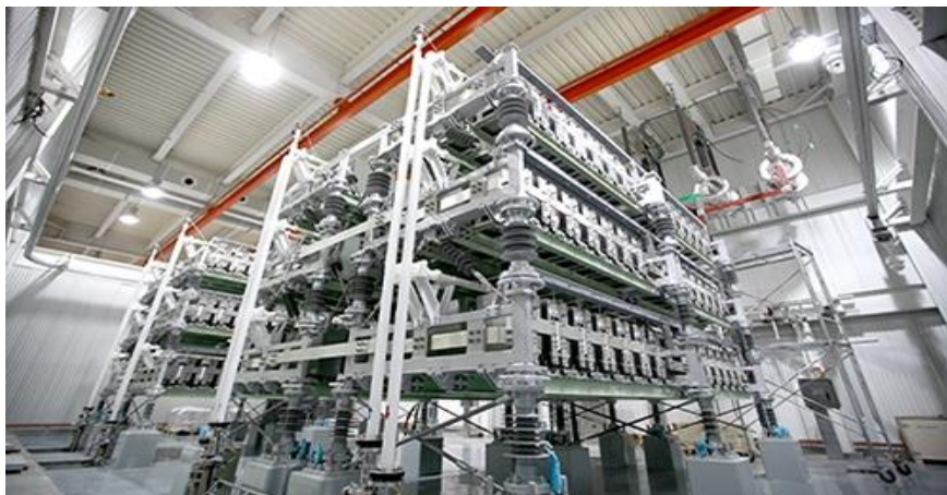
Figure (II.12): Unified Power Flow Controller (UPFC)
