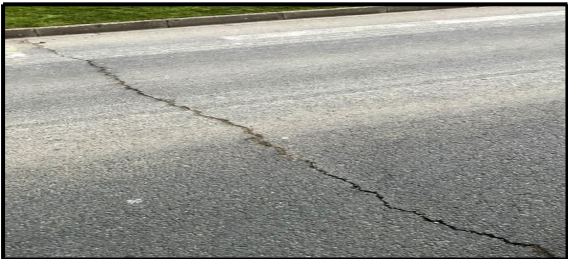
Figure II-7 : Fissure Transversale [16]
