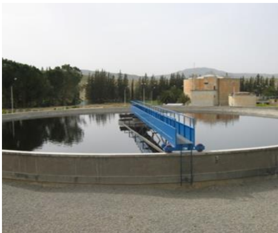
Figure I.10: ouvrages de clarification
