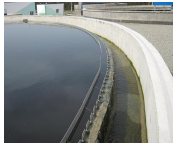
Figure I.10: ouvrages de clarification
