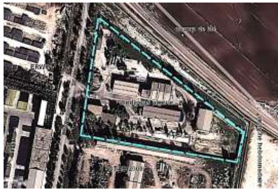
Figure III-12:Aerial view of acetylene gas industry site located in Sidi Belabes
