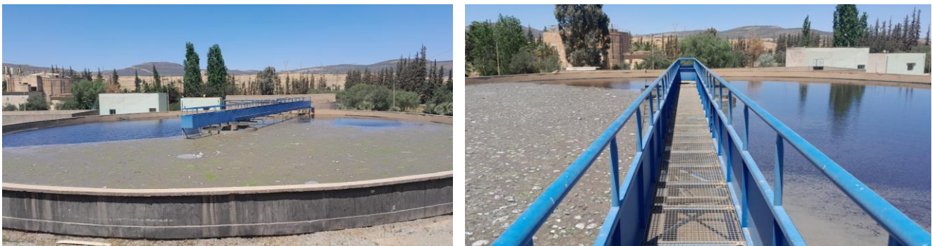
Figure II.10 : Décantation – Clarification
