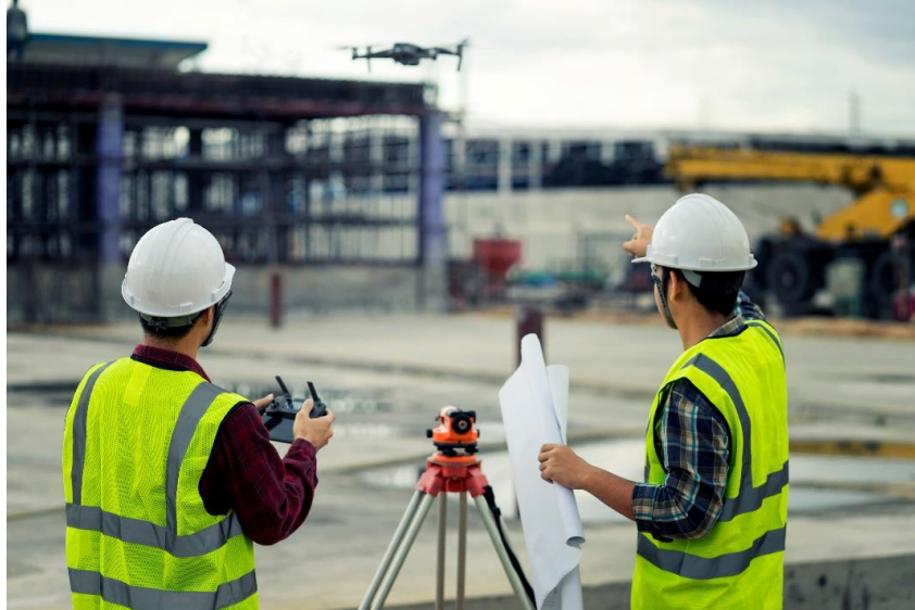
Figure 2.6. A drone takes photos of a construction site from the sky. A single flight can show the whole large site, so managers receive up-to-date information at low cost [41].
