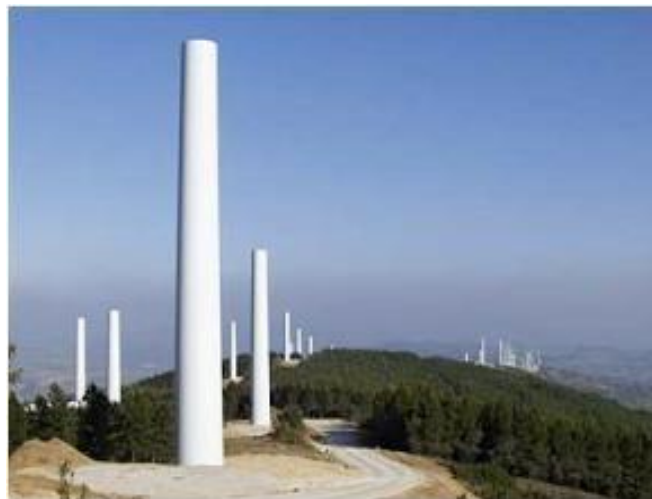
Figure I.9: Tubular Tower
