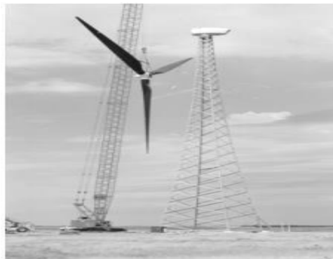
Figure I.10: Lattice Tower [14]
